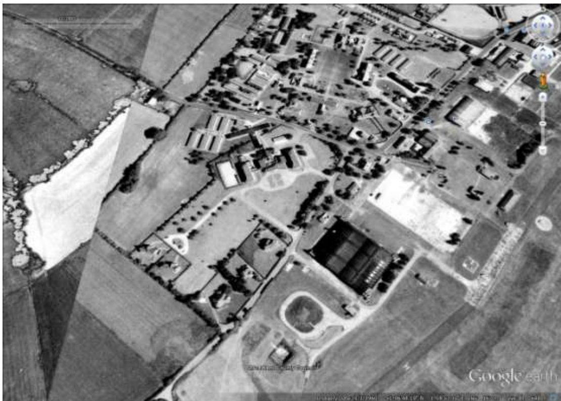
Plate 2. Google Earth dated 1960 showing almost in 3D the buildings on the PDA
